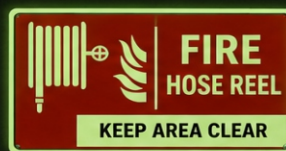
FIRE HOSE REEL
